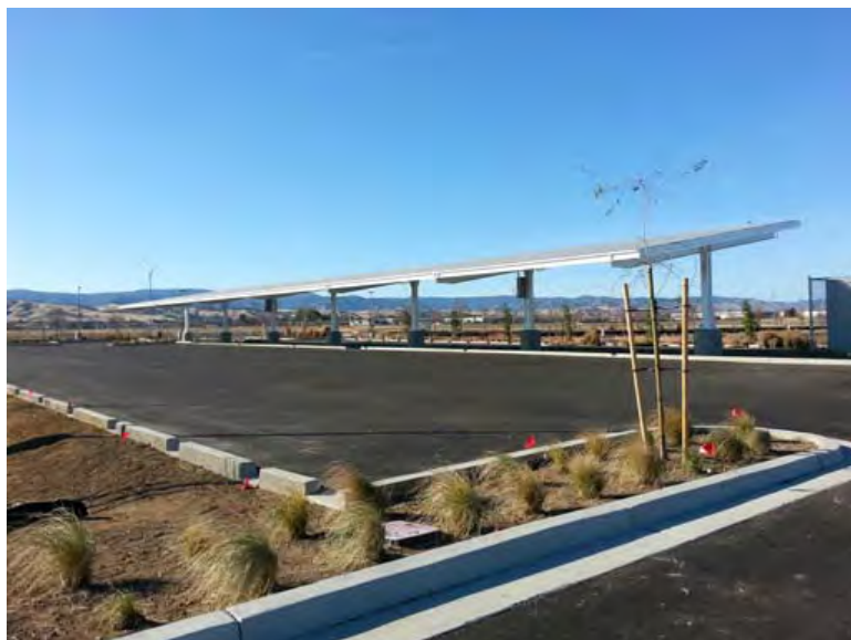
Completed parking lot area with solar panel row
